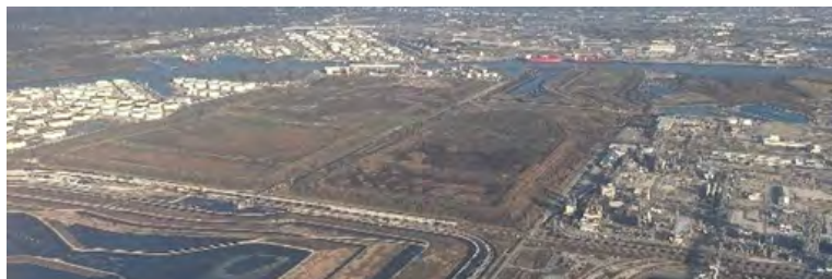
View from my flight, descending in Houston, TX: Large storage silos and petroleum extraction equipment.
